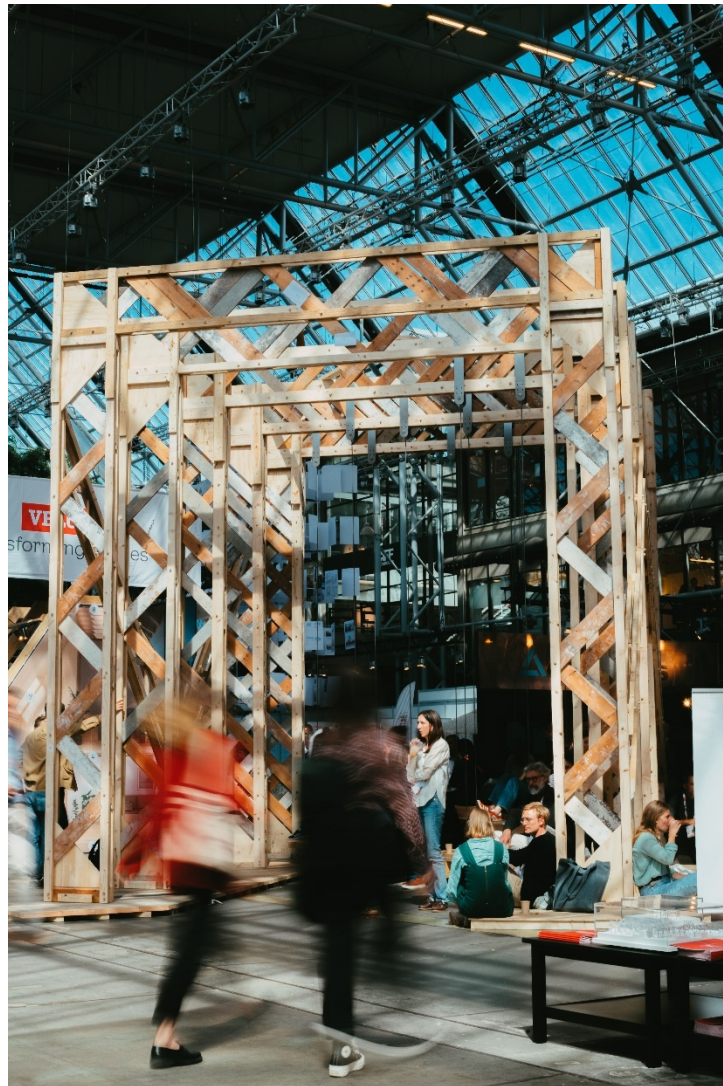
Figure 5: Complete pavilion structure with 5 frames and a hanging amphitheater
