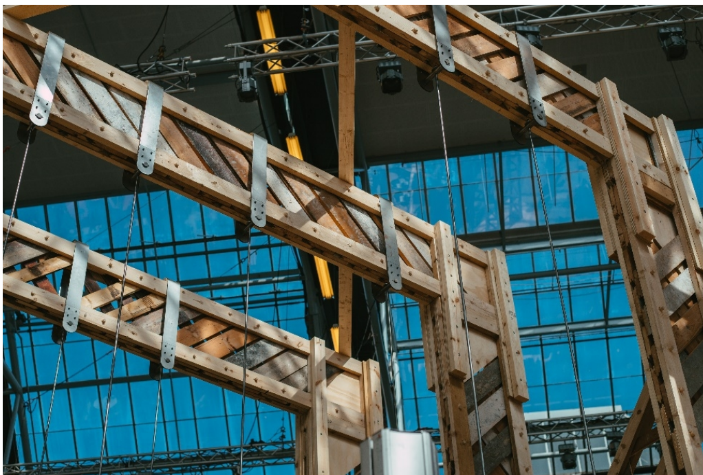
Figure 7: Steel connections that support the hanging amphitheater
